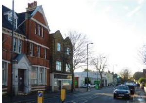
Three storey brick building (to the east side)
